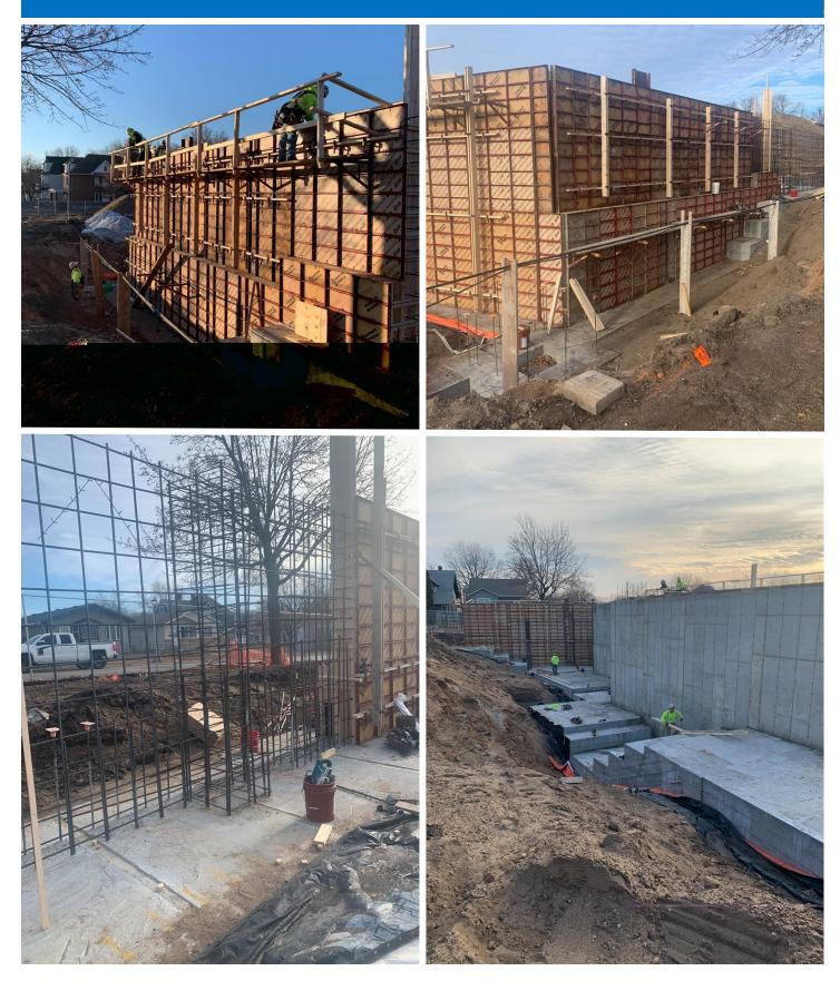
Top row: Framing up the wall panels; Second row: Rebar for wall panel; wall poured (December 2023)
